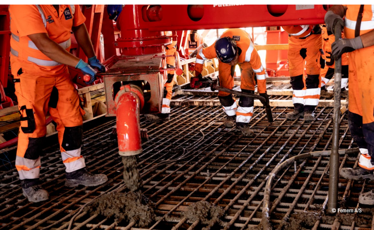
Pouring the bottom of the tunnel with the SV 7-3 swivelling distributor
